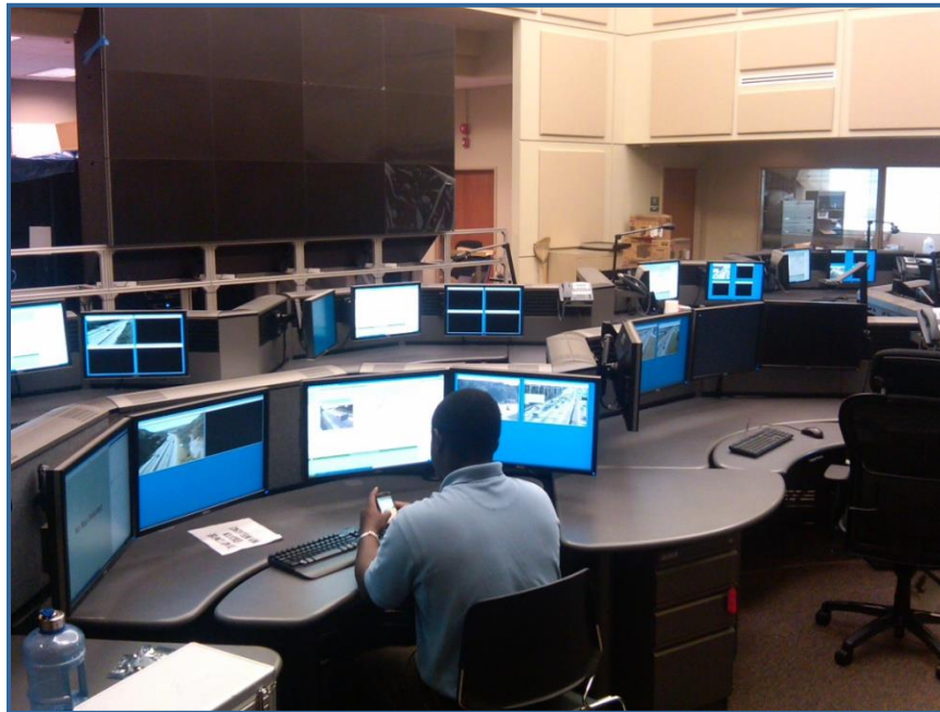
Figure 19: Cubed TMC Video Wall under Construction
